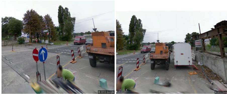
(c) Photo 4 at location B (intersection)
